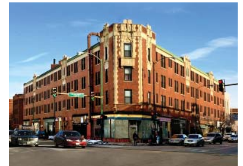
2799 N. Milwaukee – 99 Units Renovated
