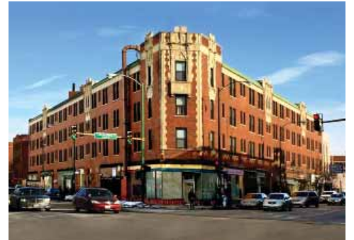
2799 N. Milwaukee – 99 Units Renovated
