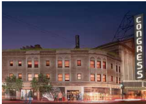
Congress Theater – $55M Renovation
