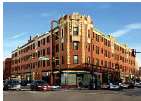
2799 N. Milwaukee – 99 Units Renovated
