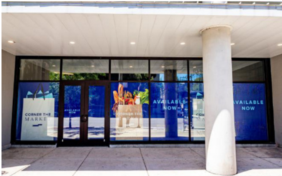
▲ Retail E - ±1,366 SF space with Milwaukee Avenue frontage
